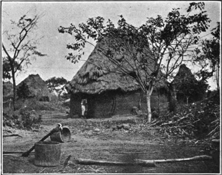
FIG. 3.—View of Smelting Houses. In the foreground are two wooden mortars and a number of pestles used for pounding the ore.
